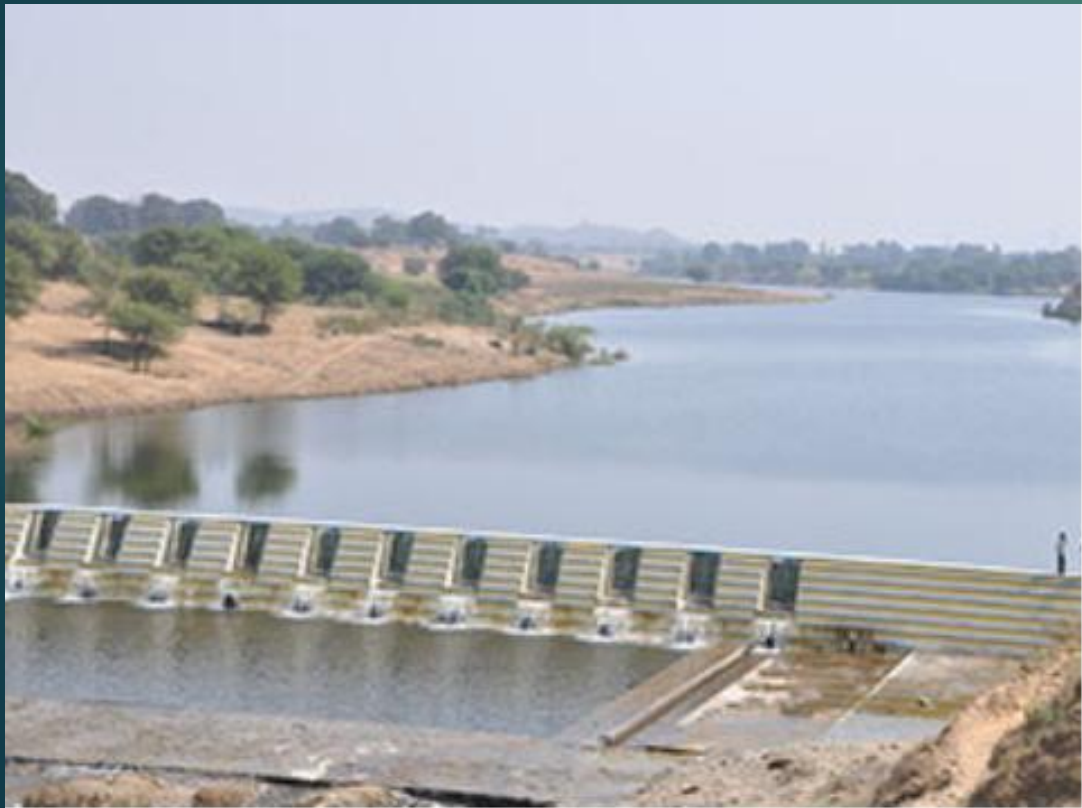
Simalaghasi Check Dam Gates across river Panama in Devgad, Dahod District, Gujarat
