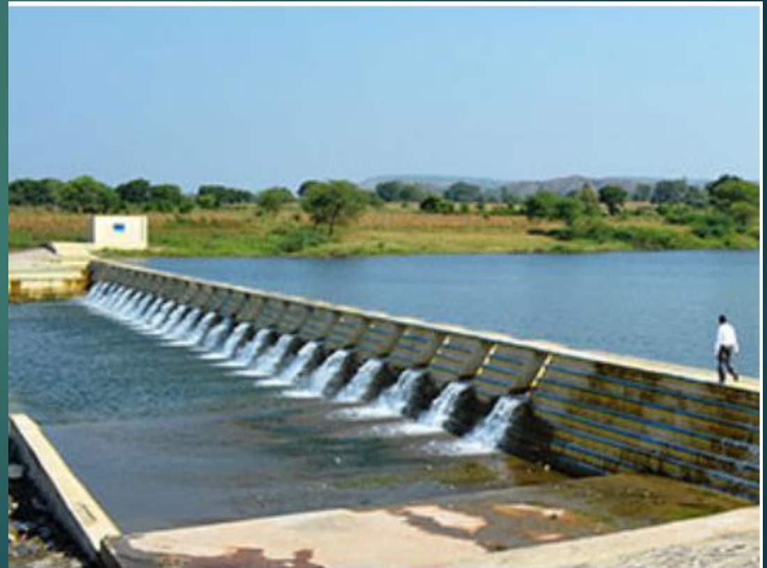
Borbhathod Check Dam Gates across river Hiren in Sajjangarh Taluk, Banswara District, Rajasthan
